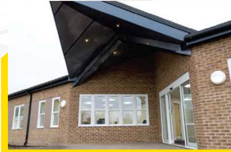
Shaw Primary Academy, Admin block.
