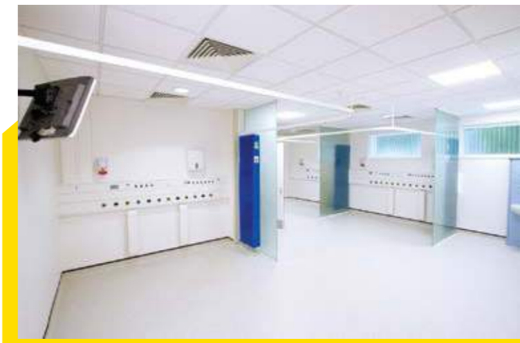
Highgate Private Hospital, Recovery suite.
