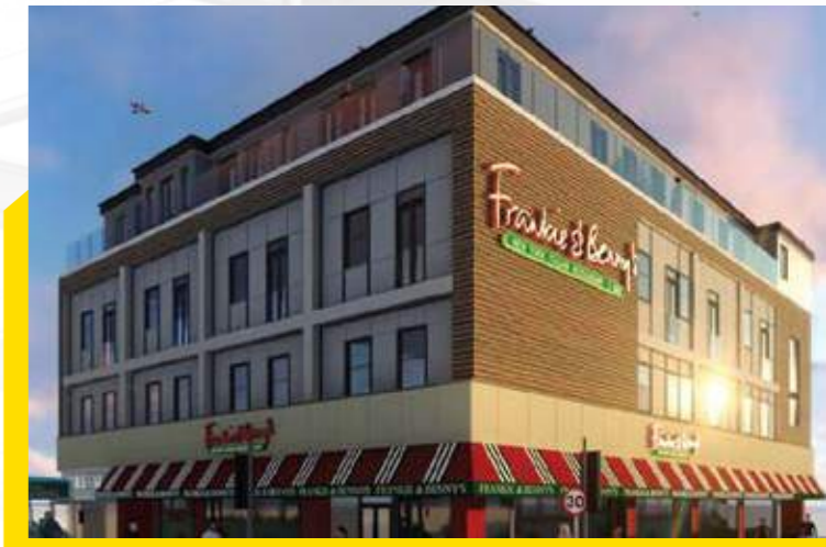
Flat conversion, Southchurch Road
